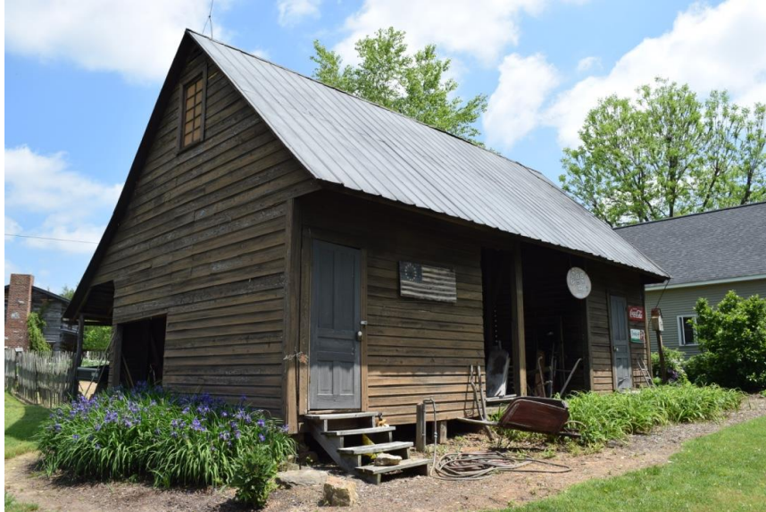
Granary, view NE
