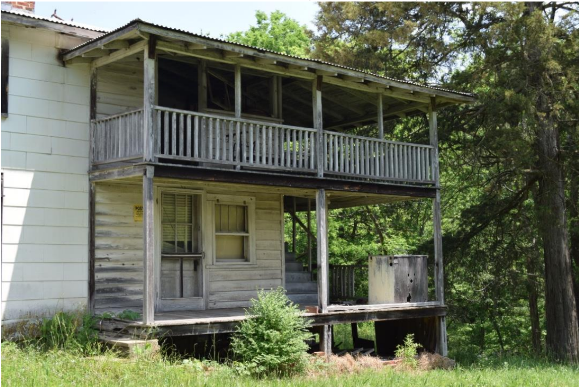
Alonzo Miller Roadside House, rear portion of west elevation, view NE
