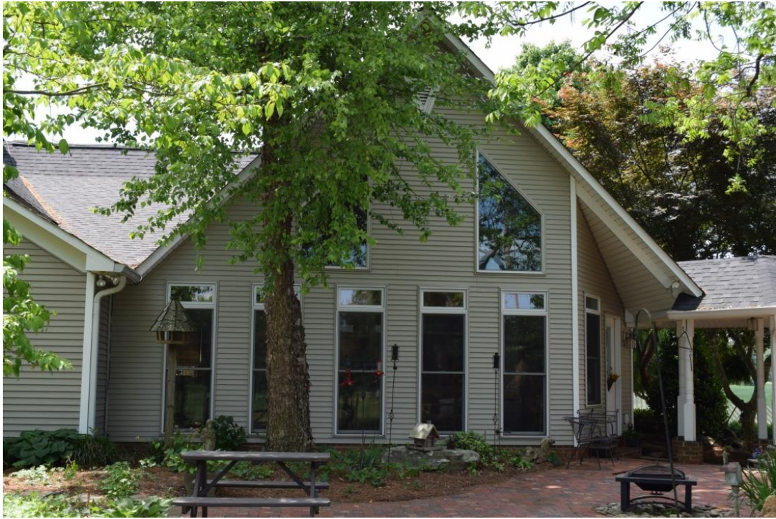
Henderson Rogers House rear elevation, view S
