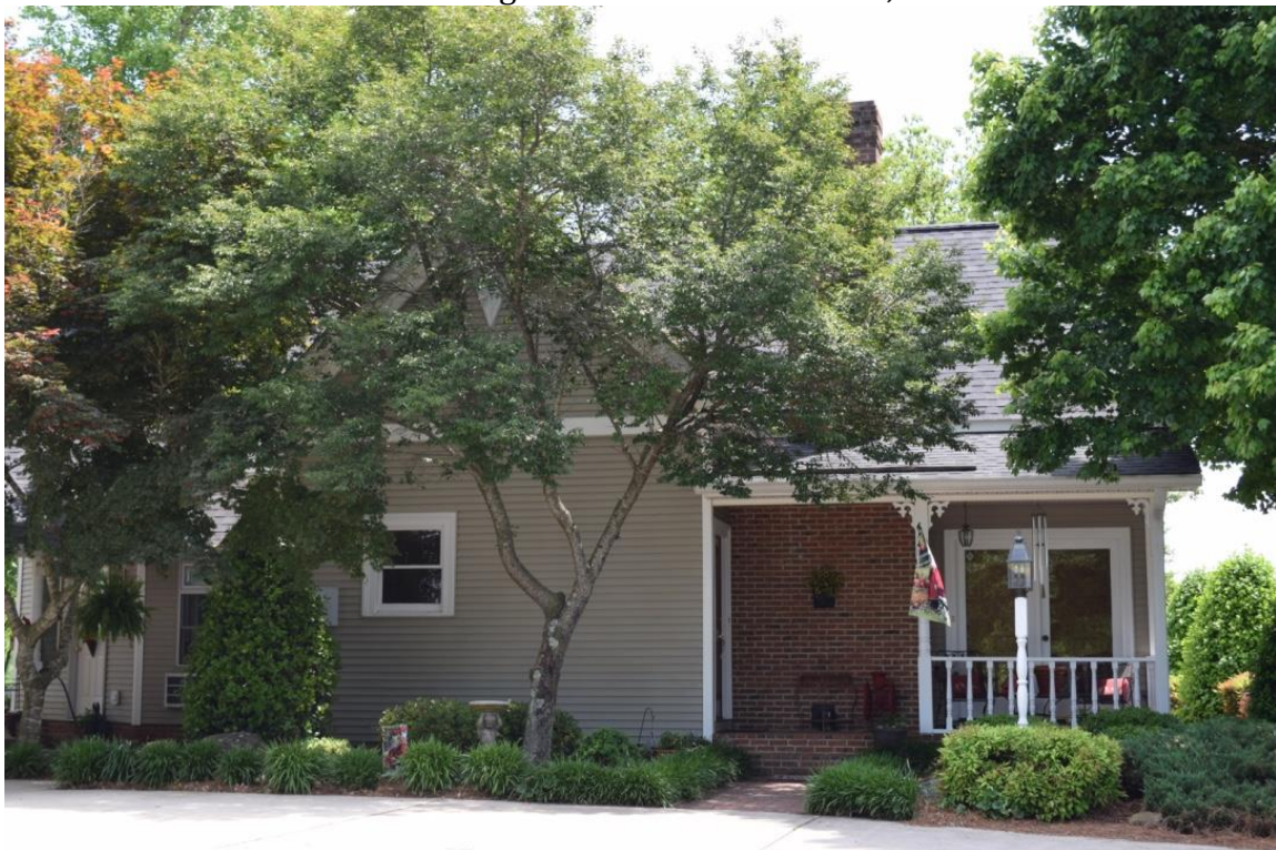
Henderson Rogers House west side elevation, view E
