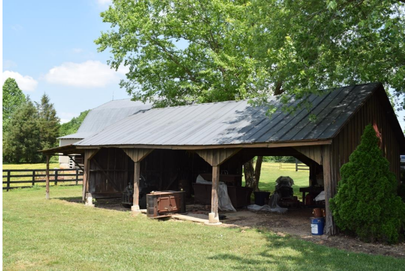
Equipment shed, view NW
