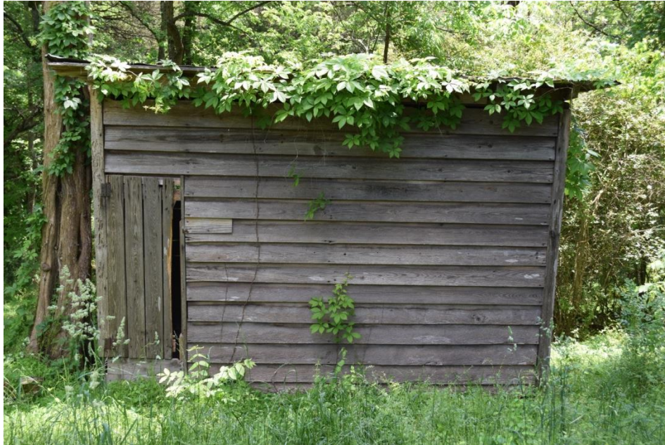
Shed, view SE
