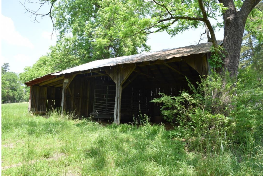
Equipment Shed, view N
