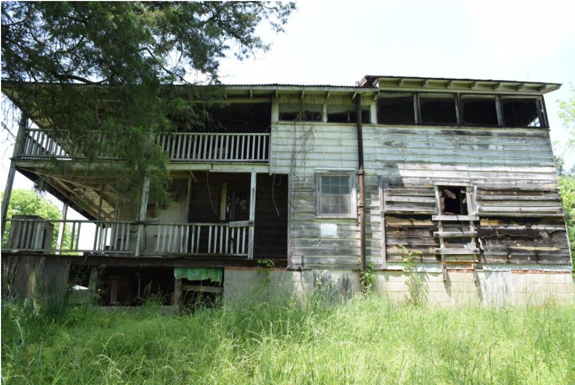
Alonzo Miller Roadside House, rear elevation, view NW
