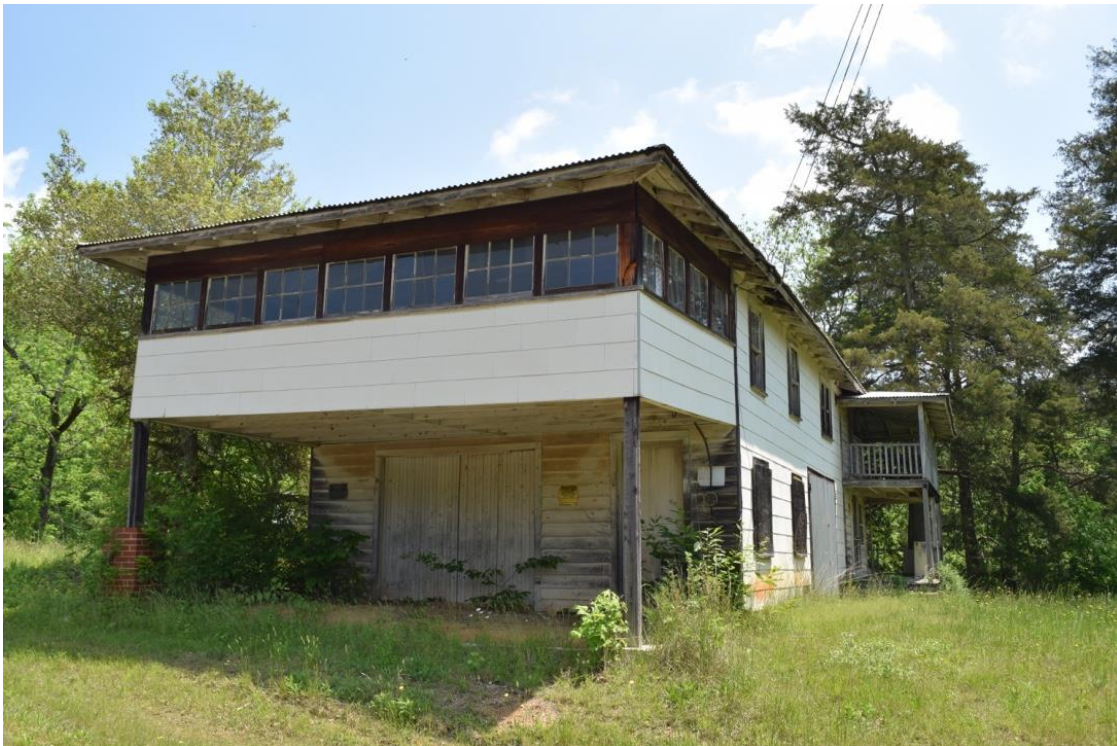
Alonzo Miller Roadside House, view SE
