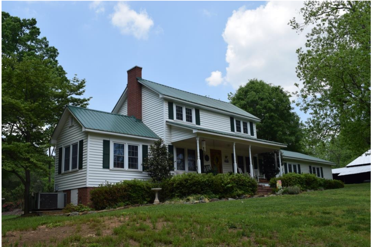
Miller House façade, view NE
