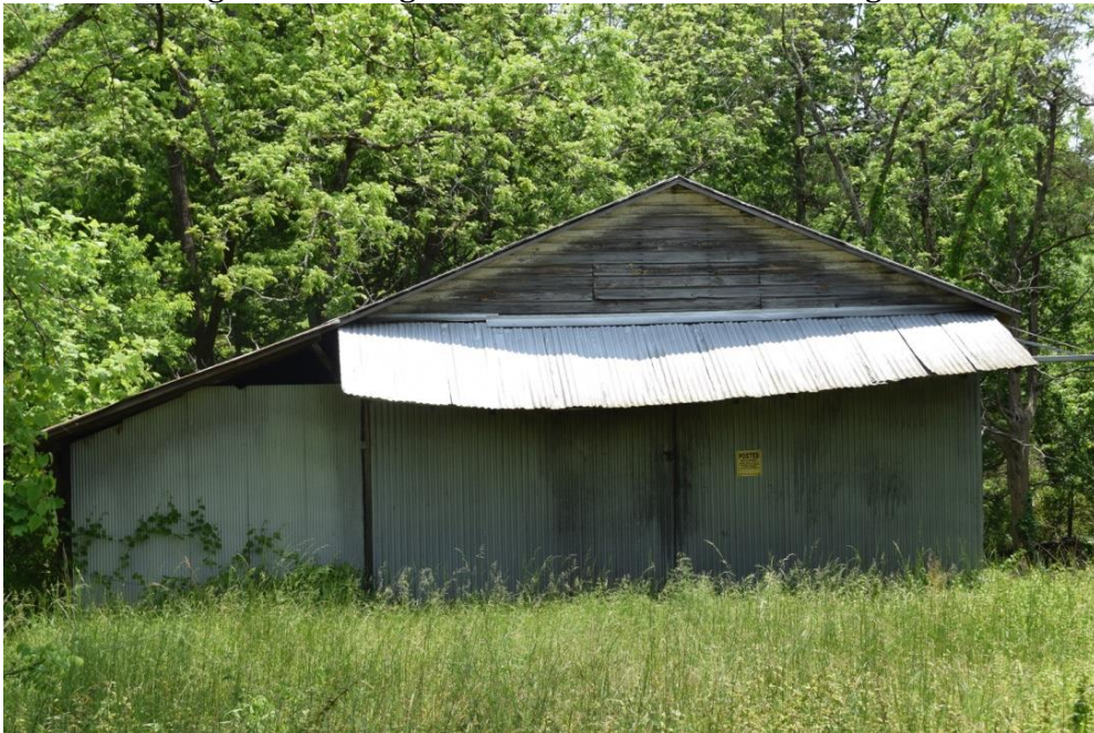
Garage/Tractor barn, view SE
