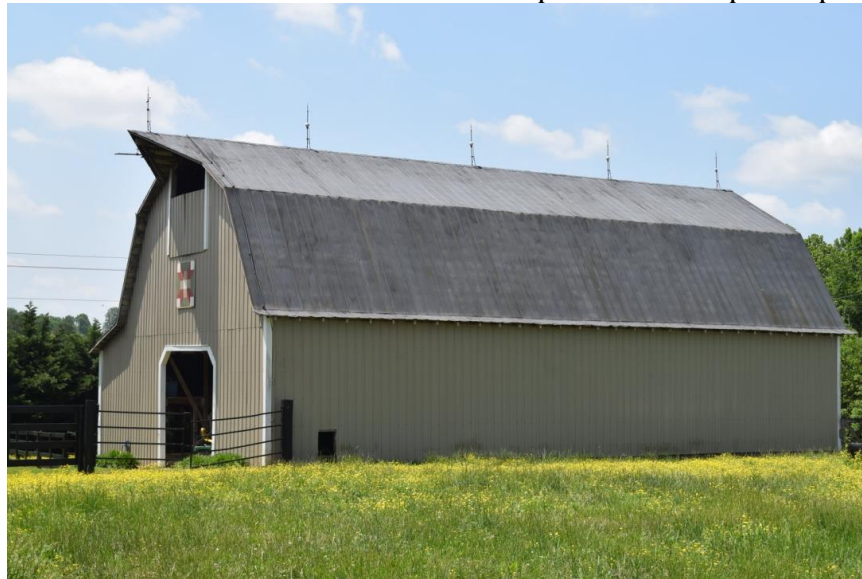
Barn, view SW
