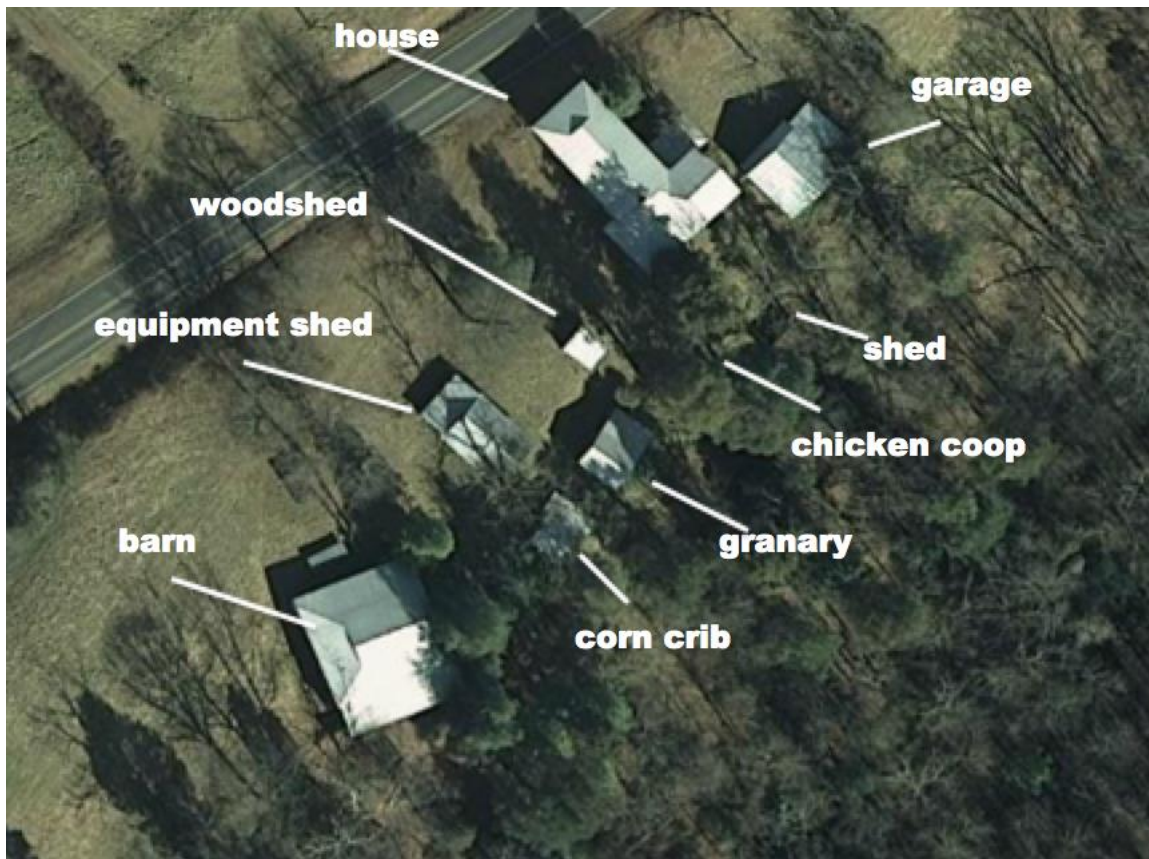
Alonzo Miller Roadside House aerial view and buildings' locations
