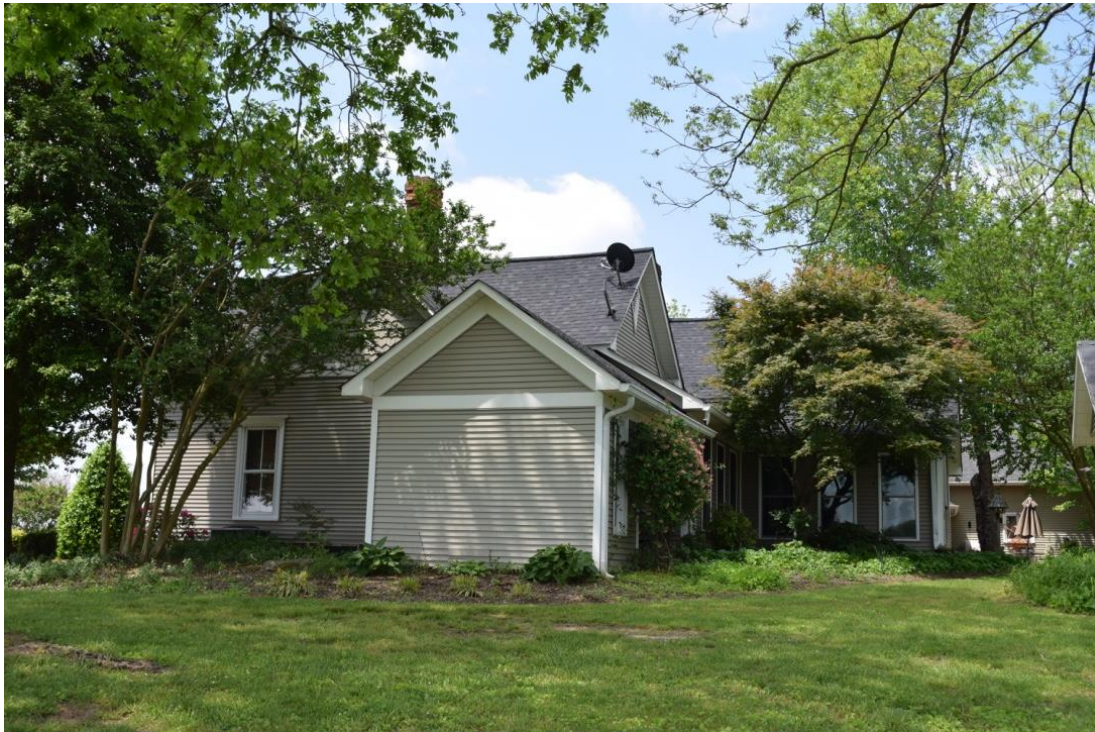
Henderson Rogers House east side elevation, view W
